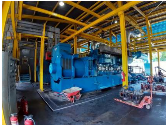
Gambar 2. 1 Diesel Generator PLTD Legon Bajak
