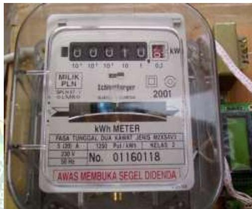
Gambar 2.3 KWH Meter Analog
