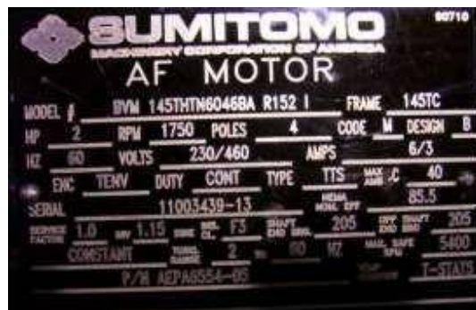
Gambar 4.16 Nameplate motor coal feeder PLTU Tanjung Jati B unit 1 & 2
