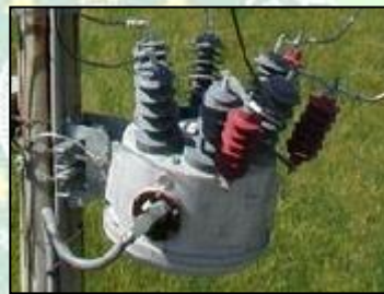
Gambar 2.17 VCB ( Vacuum circuit breaker )
