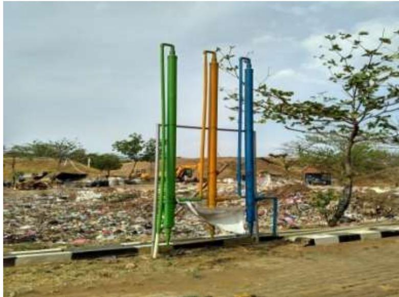
Gambar 2.8 Pipa Instalasi Gas Metan
